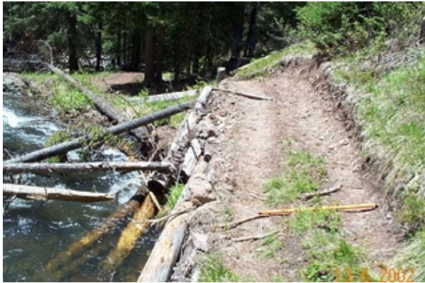
Poorly designed trail degrades water quality. Wild Trails file photo
